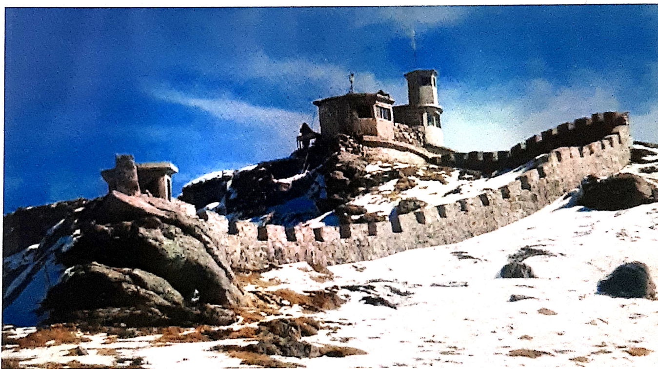
The Peoples Liberation Army post at Natu La under vigil by the Indian soldiers
